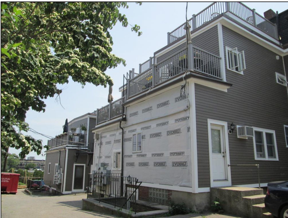
Fig. 8 View of rear extensions from Fenwick Street showing new window and a/c openings, roof decks, and in-process installation of cement board and composite trim.
