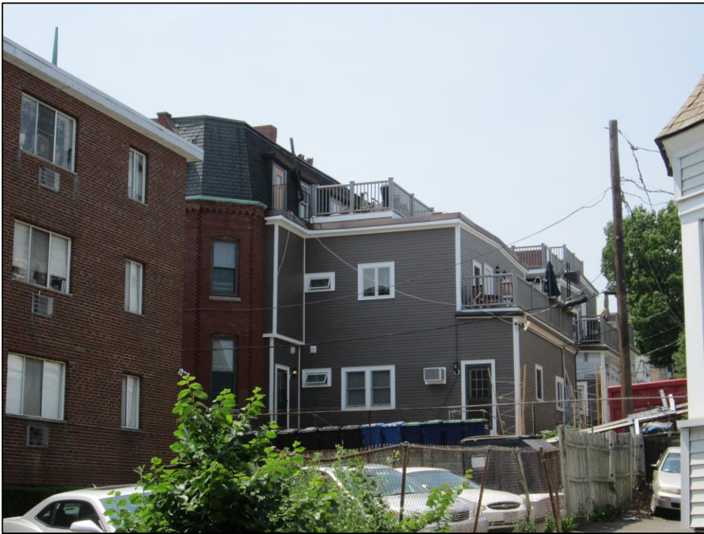
Fig. 7 Rear portion showing new window and a/c openings, new roof decks and newly-applied cement board and composite trim.
