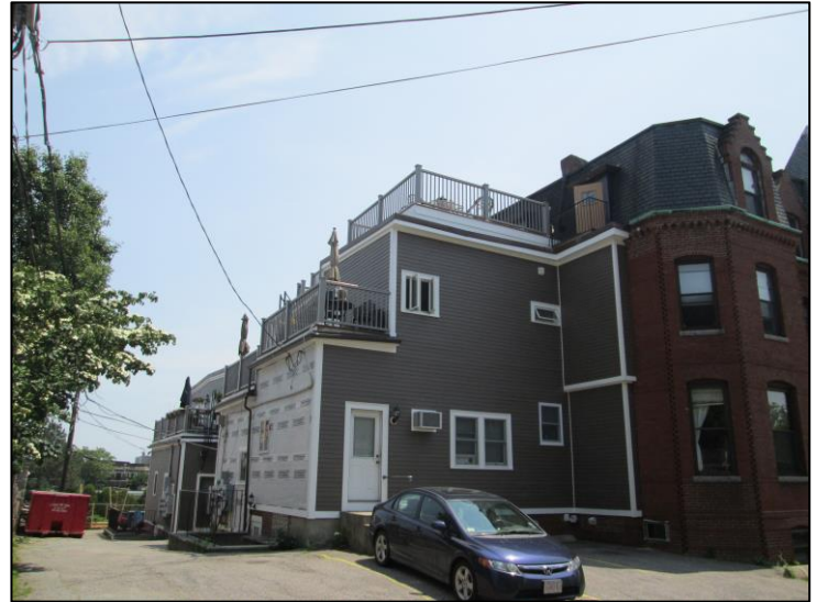
Fig. 5 Image from summer, 2015 shows project in-process with vinyl siding and wood clapboards removed and large portions of extension covered with cement board and composite trim. A/c unit opening, and large first floor window opening are new and altered in size and shape respectively.
